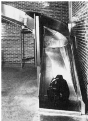
Figure 8 Chute Conveyors. (Courtesy of Standard Conveyor Company)
